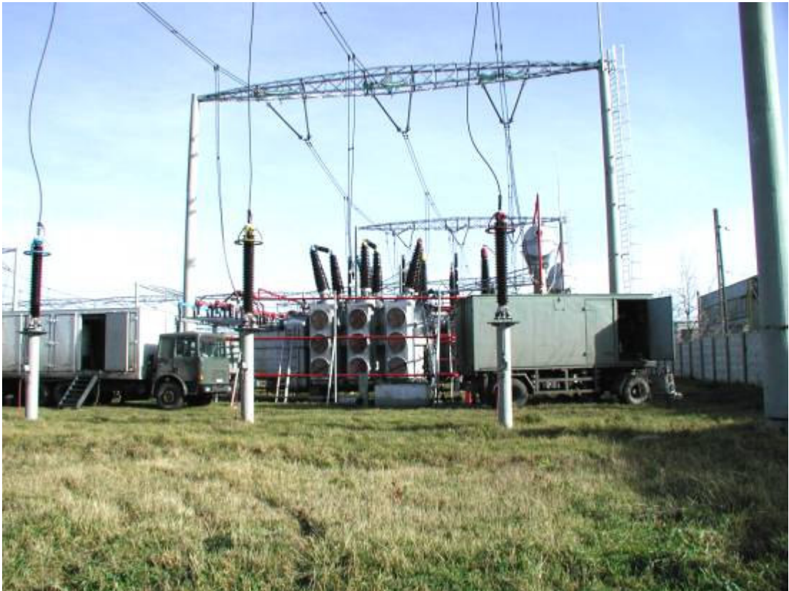
Photo 3: The insulation drying of (a+t) 400/60 MVA \pm [12 x 34,65/12] / 22kV regulating special transformer no. 85766/72, in 400 kV Sibiu-Romania substation
