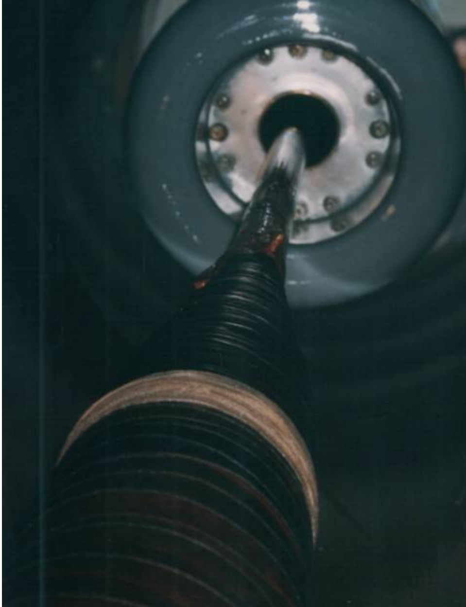
Foto 6 The control of 525 kV bushing raising from inner of the autotransformer tank
