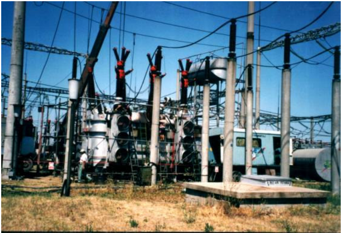
Photo 4. The insulation drying of 200/200/60 MVA 231\pm 8x1.56\%/121/20kV autotransformer no. 95731/1986, in 220 kV Turnu Magurele-Romania substation
